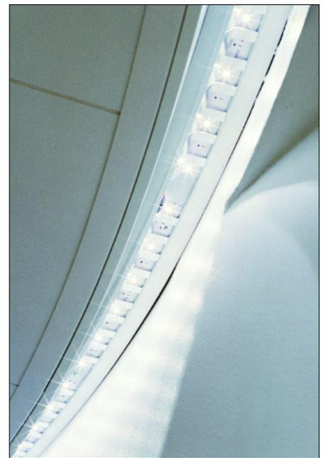
The new Turning Torso residential tower in Malmö, Sweden, is not only an architectural feat but a state-of-the-art example of modern lighting solutions. Using Golden Dragon LEDs from Osram and a custom-made fixture from the Danish lighting manufacturer Louis Poulsen Lighting, the planners of the building were able to achieve their custom installation objectives as well as implement a cost-effective and stylish lighting arrangement.
